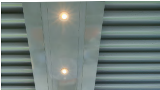
Beam Chases (Can Lights, etc.)
